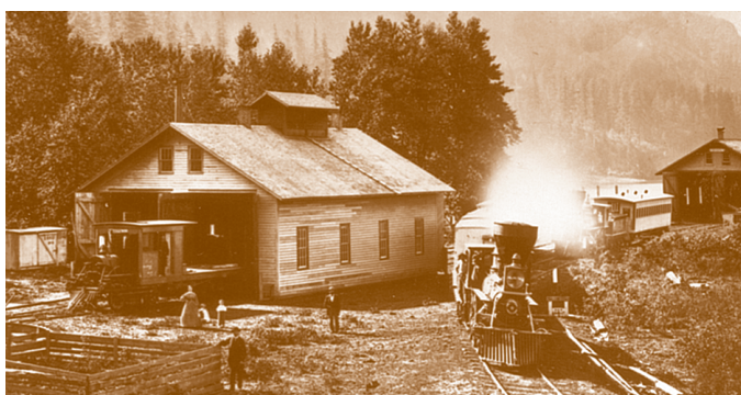
Lower Landing Terminal Facilities (1867) OHS Negative 21103, C. E. Watkins
